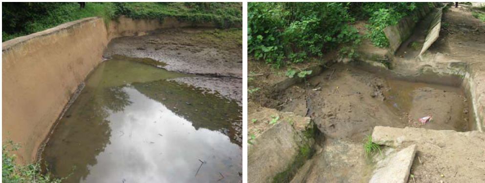
Photo 3: A section of the Ndiva storage structure (left) and a silt trap (right; Photos: Alex Oduor)
