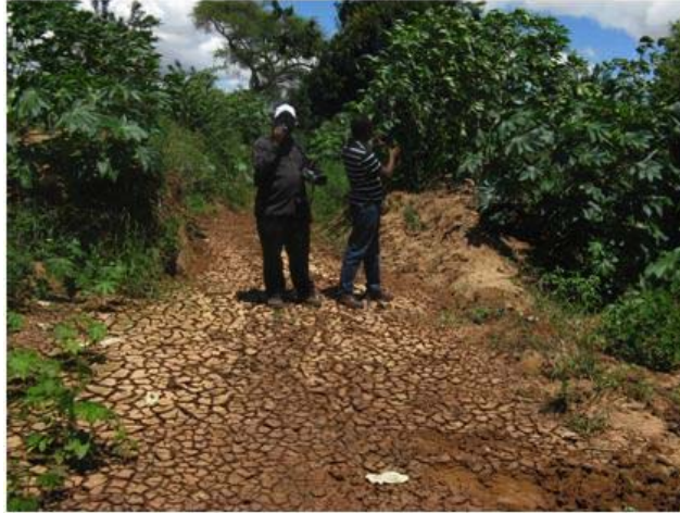
Photo 4: Canal for conveying spate water to the irrigation fields in lower Makanya catchment (Photo by Dr. Fredrick Kahimba)
