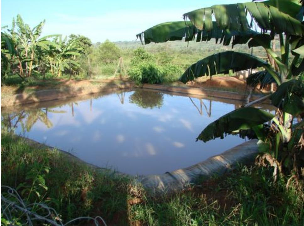
**Figure 2: Plastic lined runoff-harvesting pond in Rwanda (Photo M. M. Malesu)**
