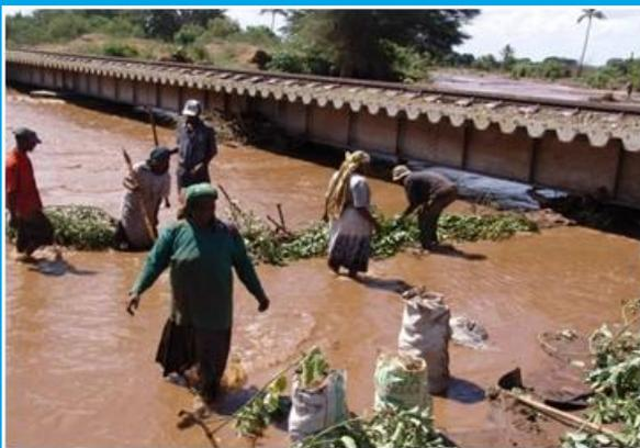
Flood water diversion WHT in Same District, Kilimanjaro Region. Water from the ephemeral rivers is normally diverted directly into the crop fields. The traditional spate irrigation structures allow some water to be diverted and some to flow further downstream.
